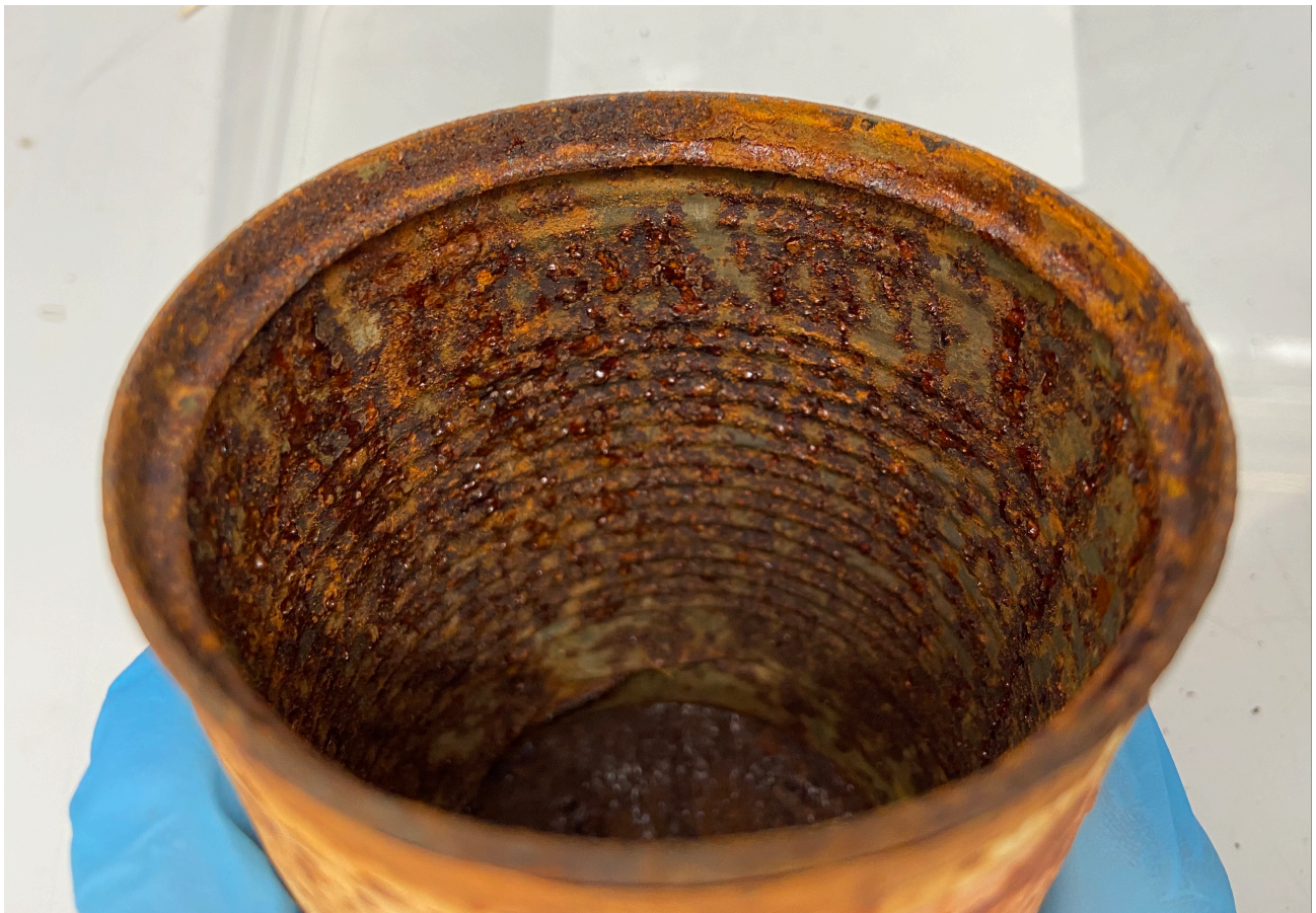
Figure 3. Detailed image of inside deterioration. Shows the areas that are not yet corroded, as well as the oil imbedded in the rust. Shows some dents in the top of the can from inside (left of the inside lid).
